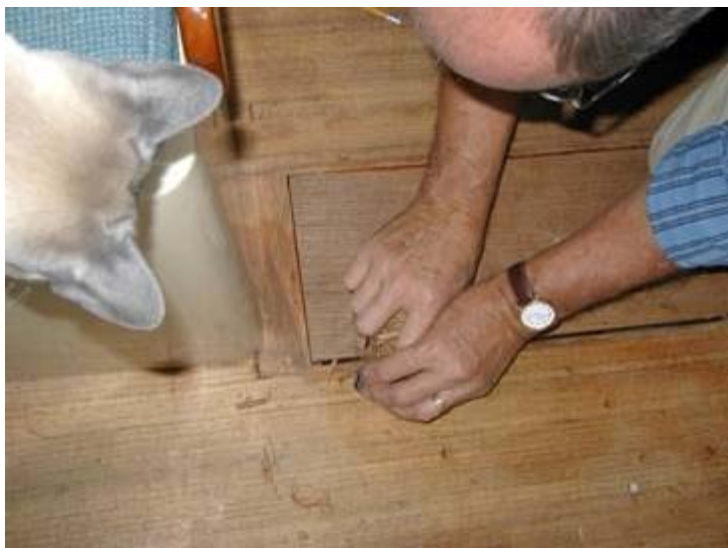
Figure 5 - Trimming the frame for a good fit while Julio the cat watches
