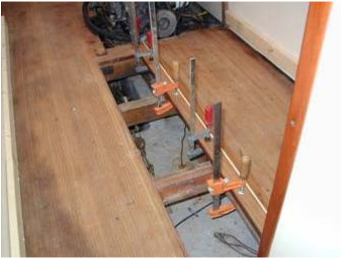
Figure 9 - Clamps are placed on the first plank
