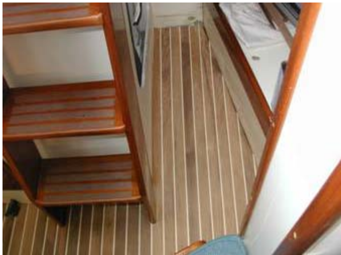
Figure 18 - Completed floor in quarter berth awaiting a coat of sealant
