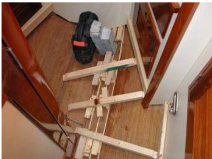
Figure 17 - Clamping braces are nailed to the old floor to hold wedges
